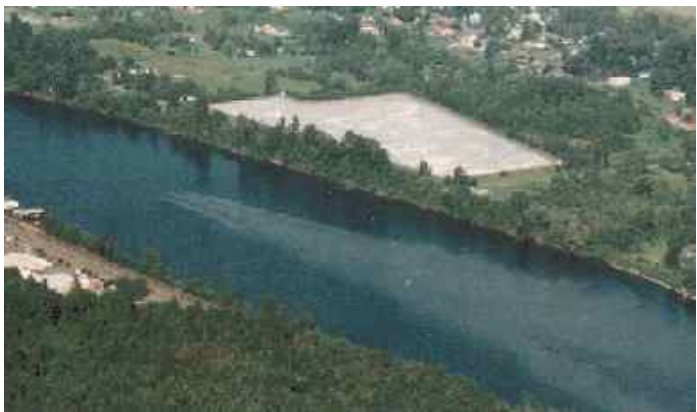
The West Linn sewage treatment plant, showing its effluent discharge into the center of the Willamette River.
