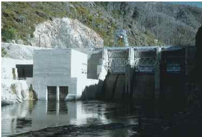
The powerhouse at Big Cliff Dam on the Santiam River.
