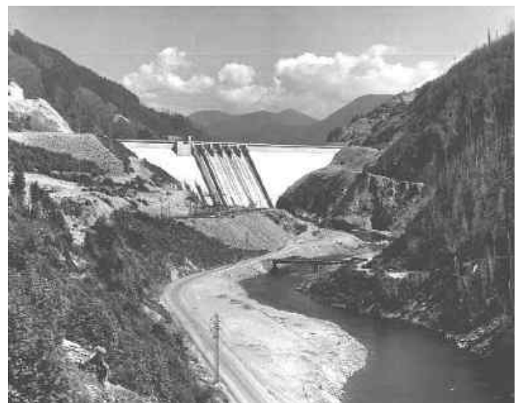
Detroit Dam, 1953. Photo: Salem Public Library Historic Photograph Database, Salem Public Library, Salem, Oregon.
